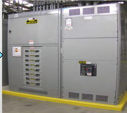
Distribution Switchboards
