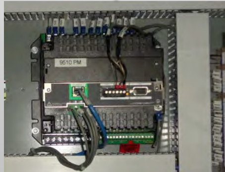
Main Breaker Meter: Siemens 9510
