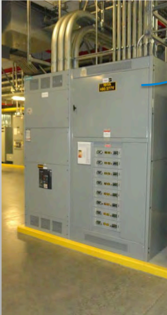
Main Breaker Meter: Siemens 9510
